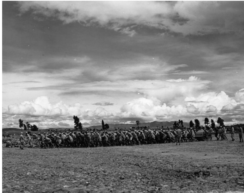
Fig 2: Chinese laborers pull a roller to smooth a runway for a B-29 airstrip. US Army 55
